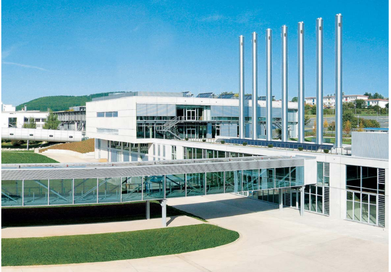
Energy centre and Viessmann Academy at the Allendorf site.
