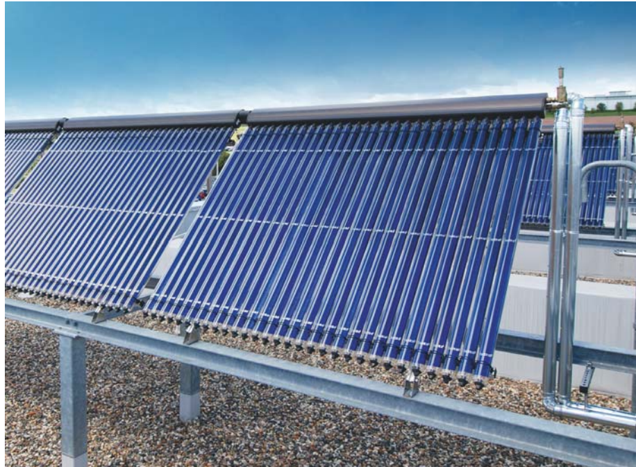
The walk-on solar roof with tube collectors delivers energy for heating in winter and cooling in summer.
