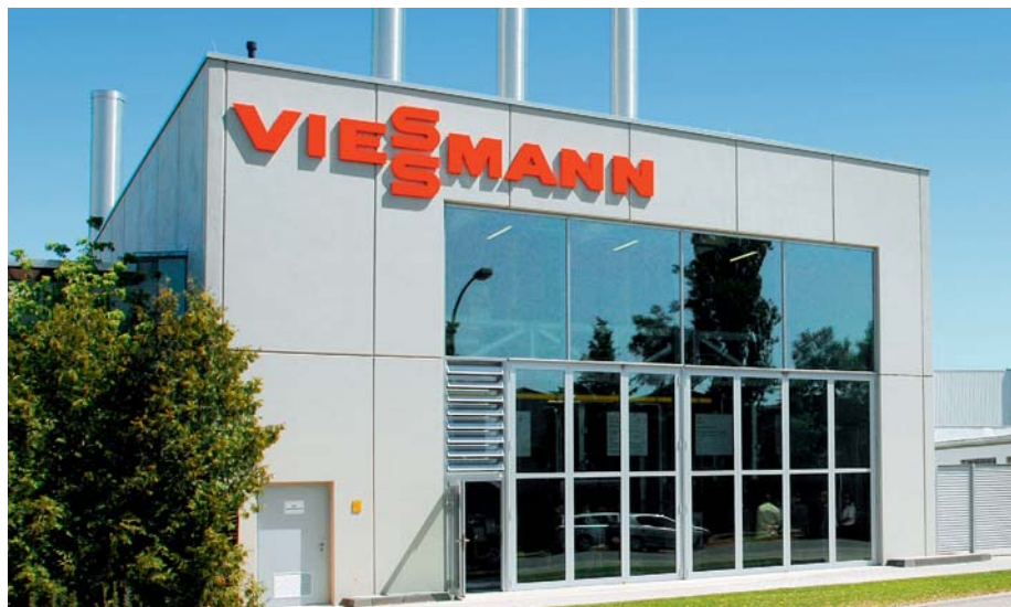
The new energy centre at the Viessmann site in Berlin.
